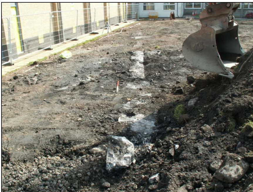
Plate 1. Stone wall 103 , view to the northeast
