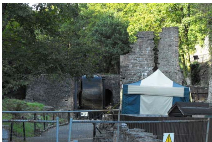
The excavation at Aberdulais Falls
