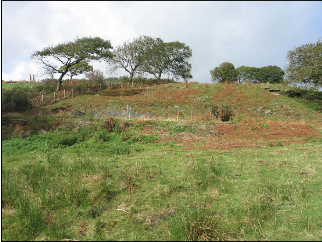
Plate 30. Building Platform E of Allt-y-Fanog, view to the N
