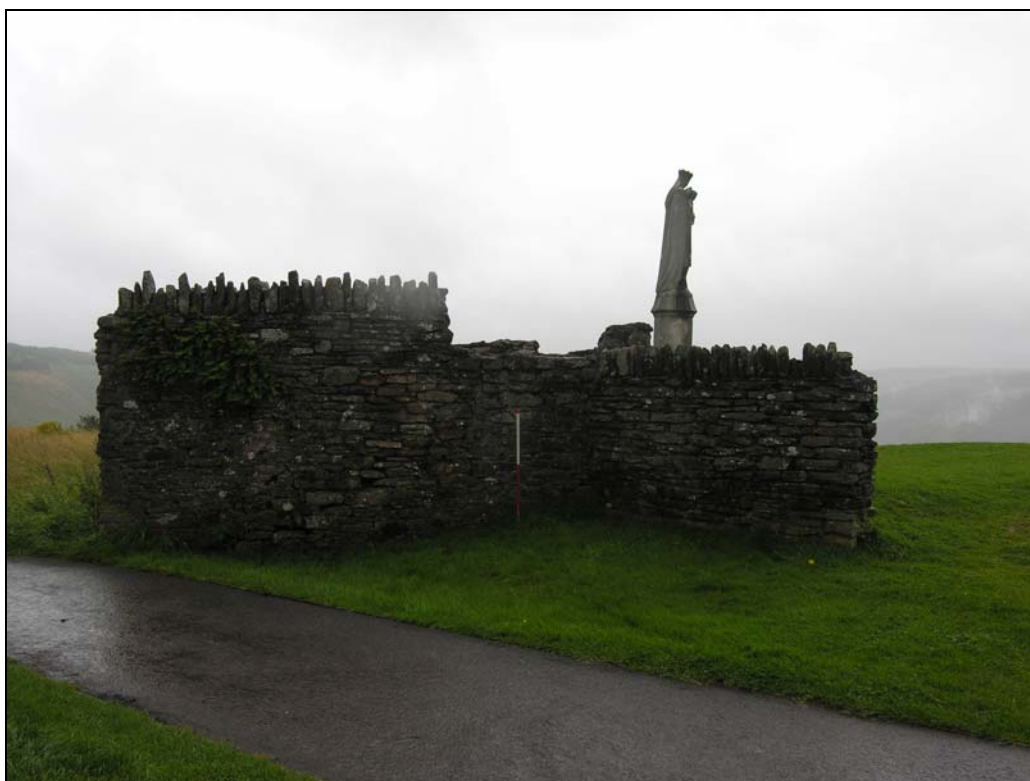
Plate 26. St Mary's Chapel, view to the SW
