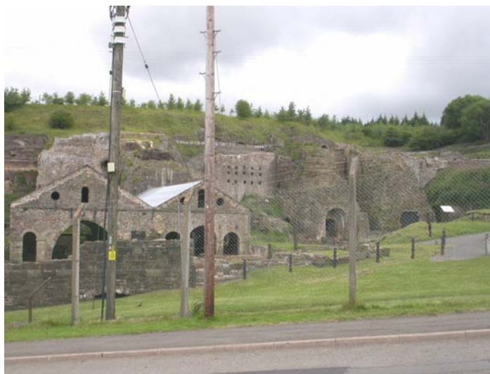
Blaenavon Historic Landscape, HLCA 006 Blaenavon Ironworks
