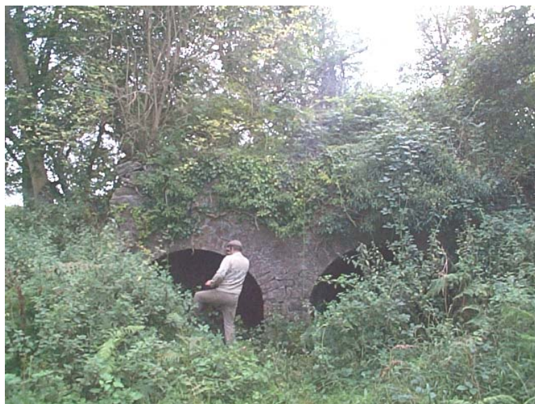
Limekiln at Penterry Farm, Nr St Arvans
