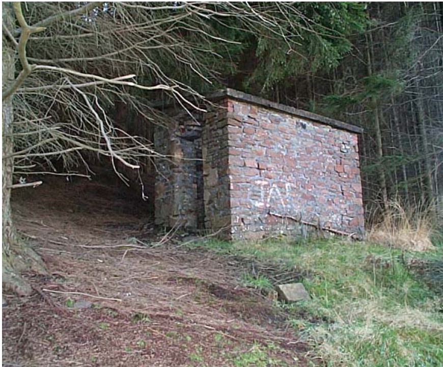
Mining explosives store at Cwmparc, NPT, to be restored
